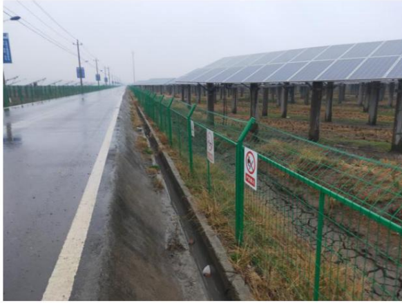
Figure 1-1 Drainage ditch in photovoltaic area
