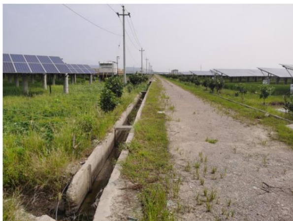
Figure 1-5 Road drainage ditch in the photovoltaic field
