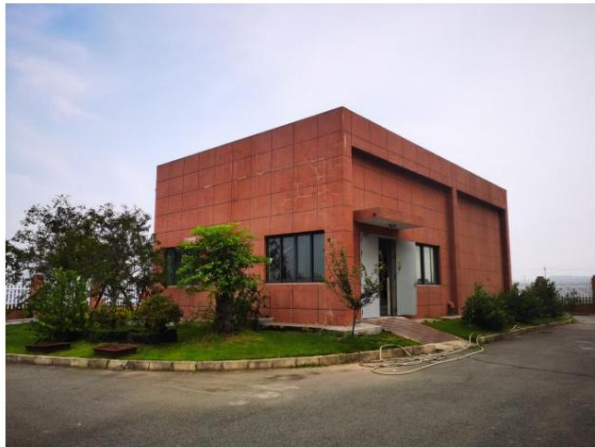
Figure 1-11 Greening in the booster station
