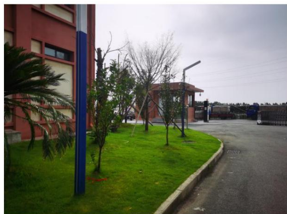
Figure 4-2 Greening in booster station
