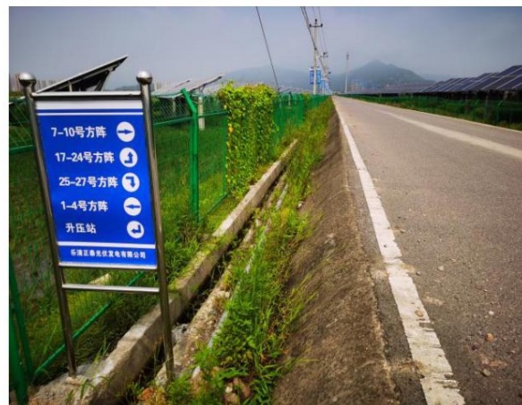
Figure 1-6 Road drainage ditch in the photovoltaic field
