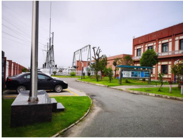
Figure 1-9 Roads and drainage in the booster station
