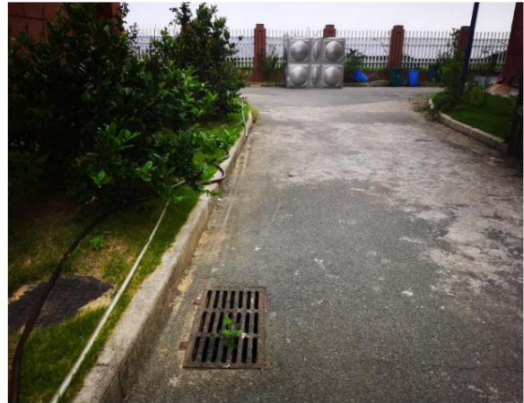
Figure 1-10 Roads and drainage inside the booster station
