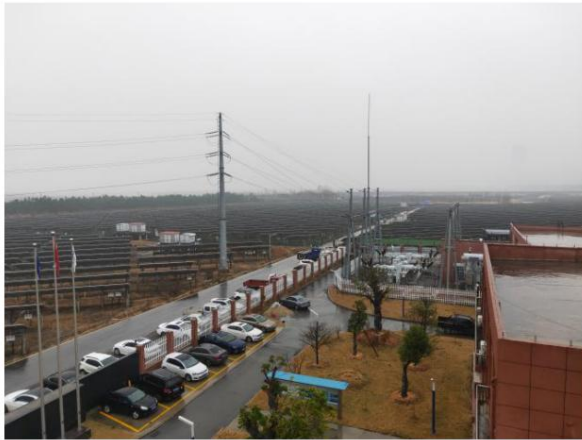
Figure 1-3 Greening of booster station
